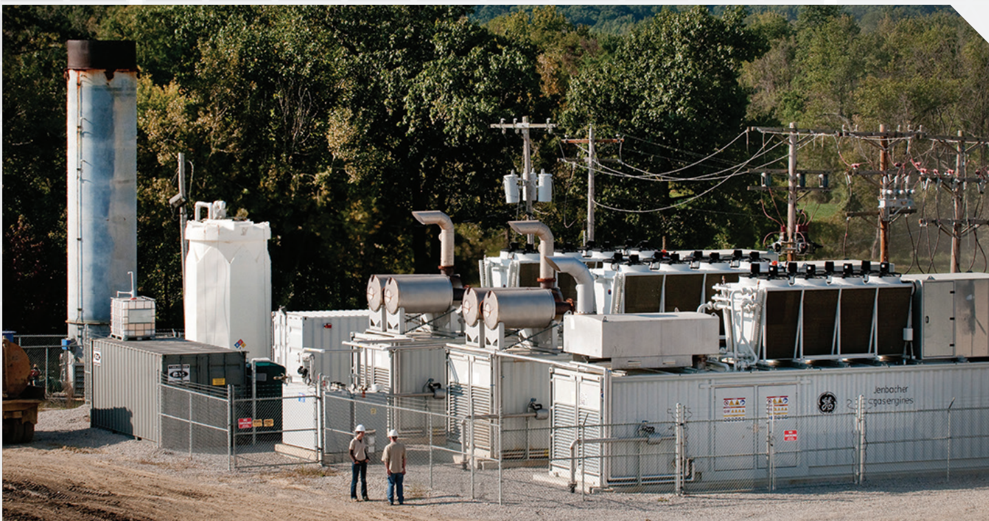
Clark-Floyd Landfill Methane Gas Plant
