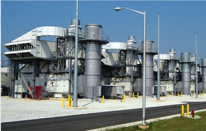
Lawrence Generating Station
