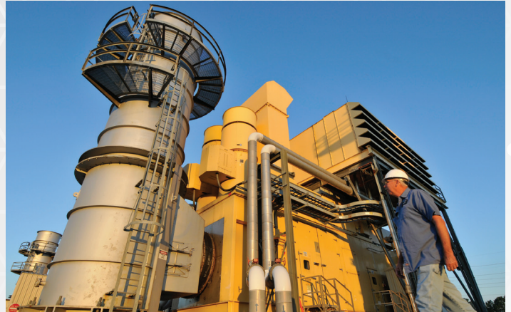
Worthington Generating Station
