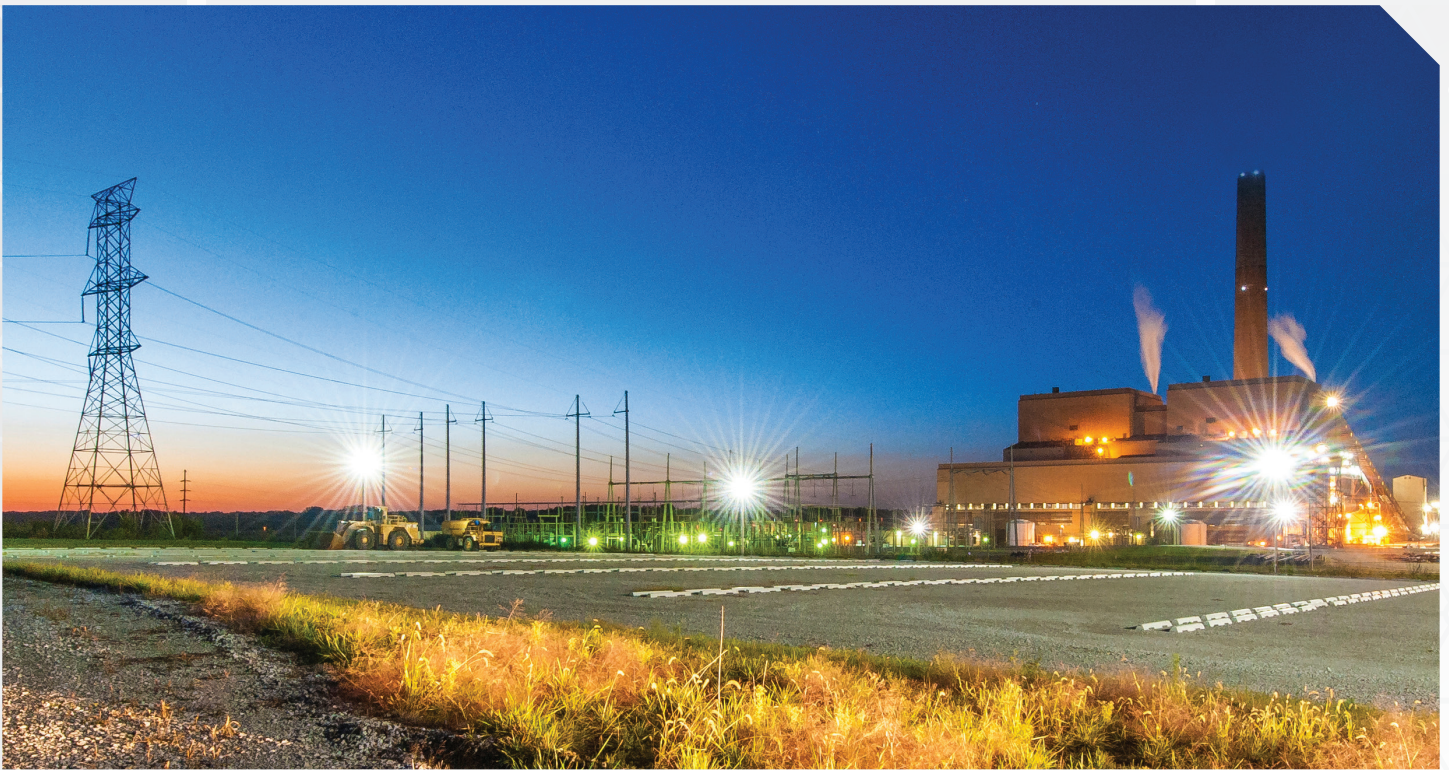
Merom Generating Station in Sullivan County
