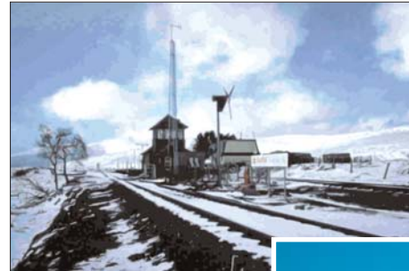
The Proven 2.5 has been powering lights at this remote station for 13 years
